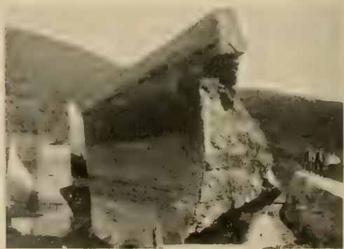
PORTION OF DAM MOVED TEN FEET
